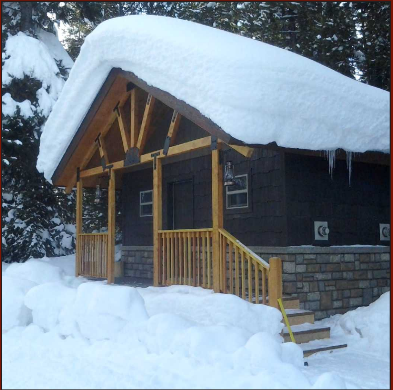
The camp bathrooms and shower facility
